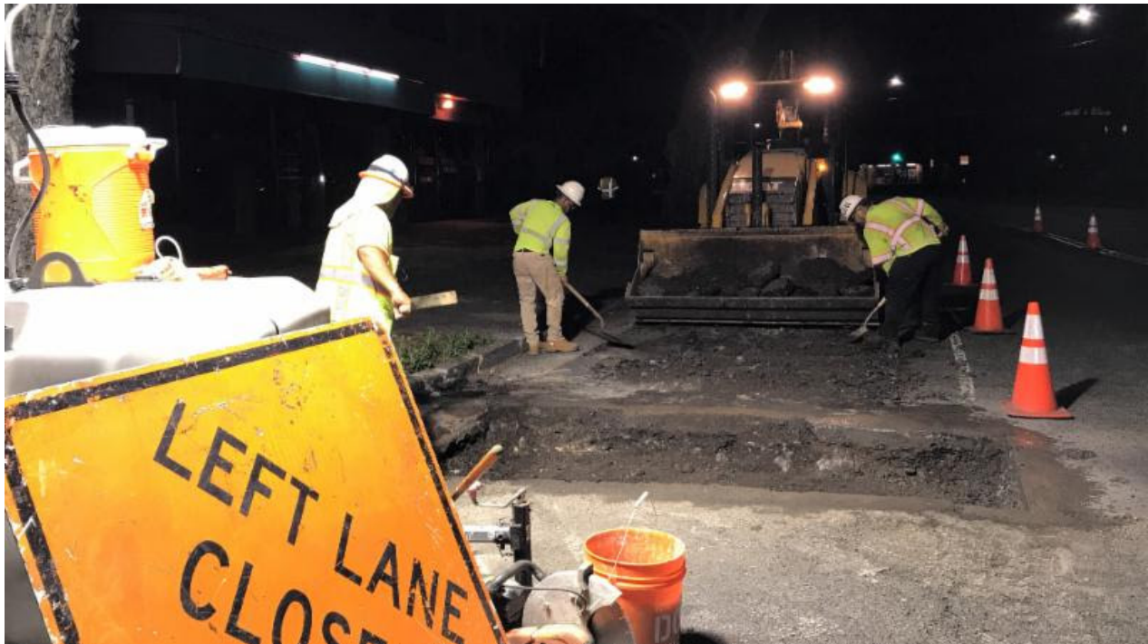
Trench patching on Dillingham Blvd.
